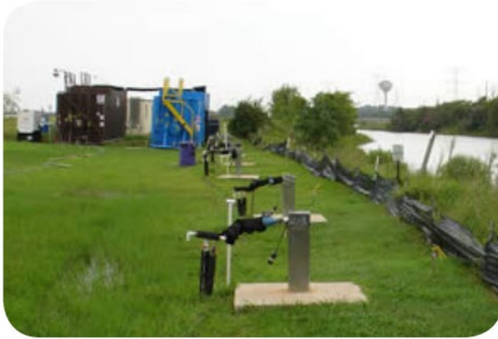
Groundwater Pumping Wells
