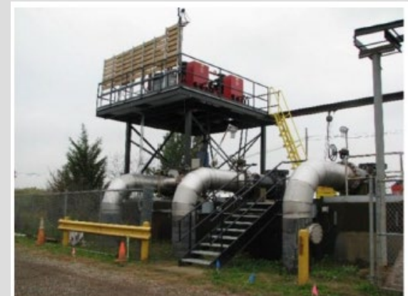
Elevated electrical controls for full-scale groundwater extraction
